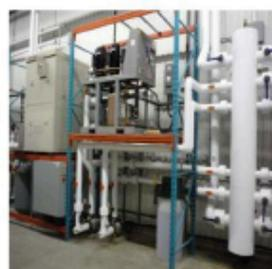
\* provides ~100 kW of process hot water at 60-75C delivery temperature
